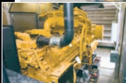
Above: Each of the 8 Caterpillar engines generates 1.3 megawatts of power.
